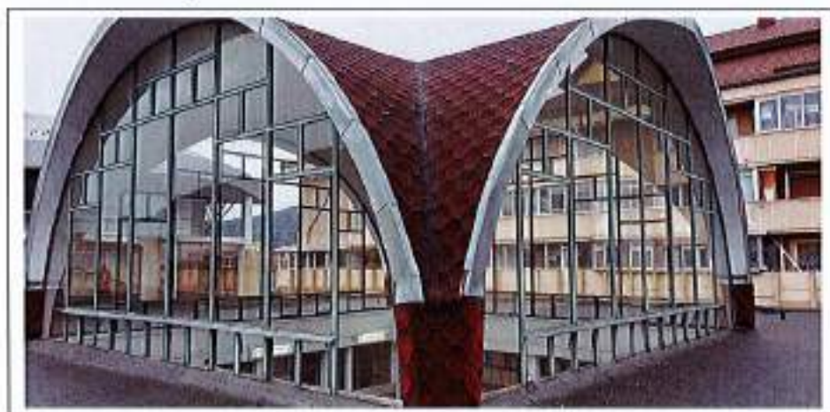
Fig. 18 - Cupola luminator (corp A)
