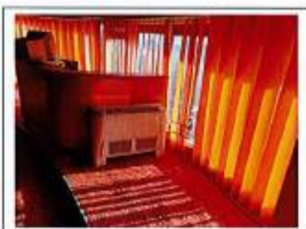
Fig. 57 Ventiloconvector amplasat in mansarda
